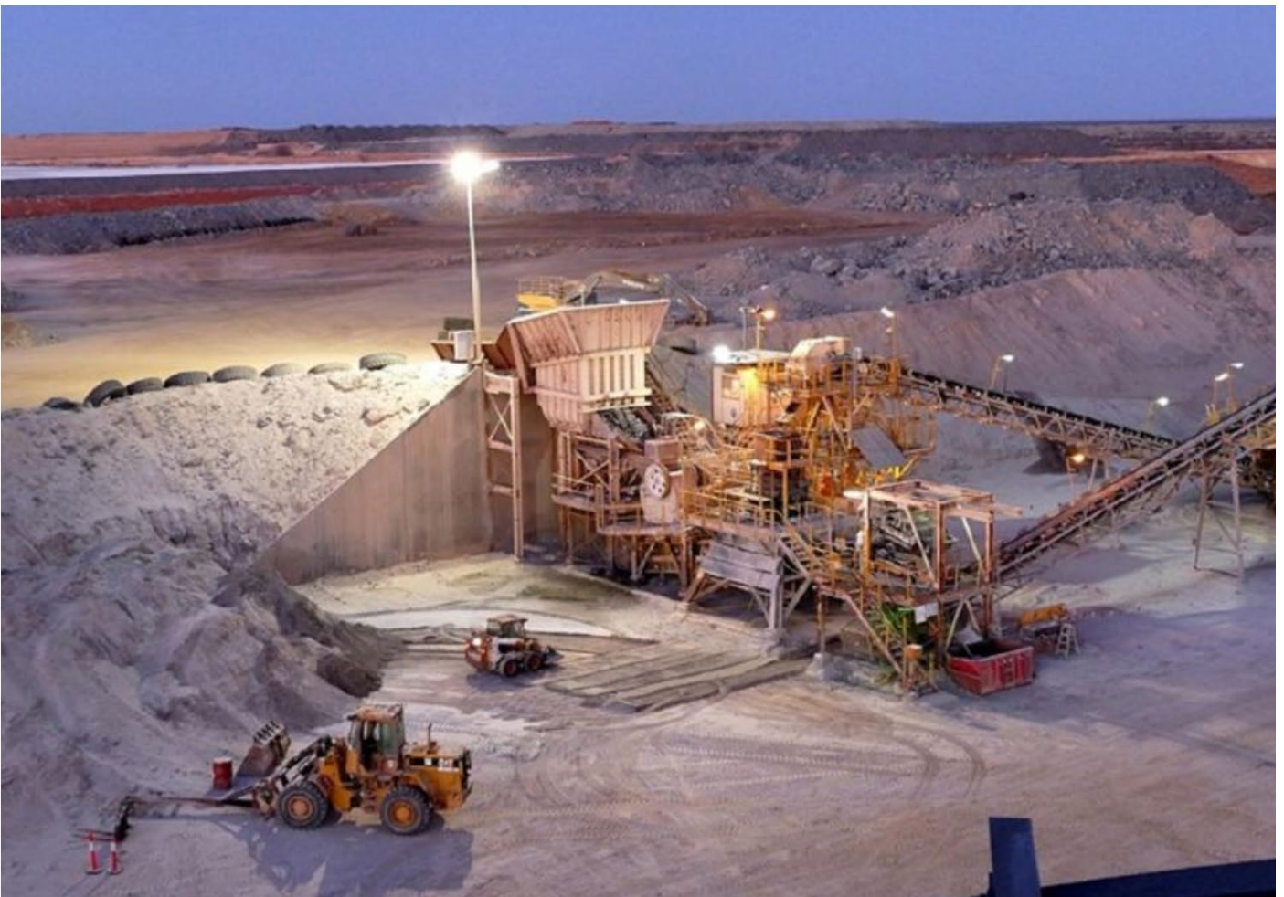
Barton Gold's crushing circuit at the Challenger gold mine in South Australia, currently on care and maintenance. Credit: File
