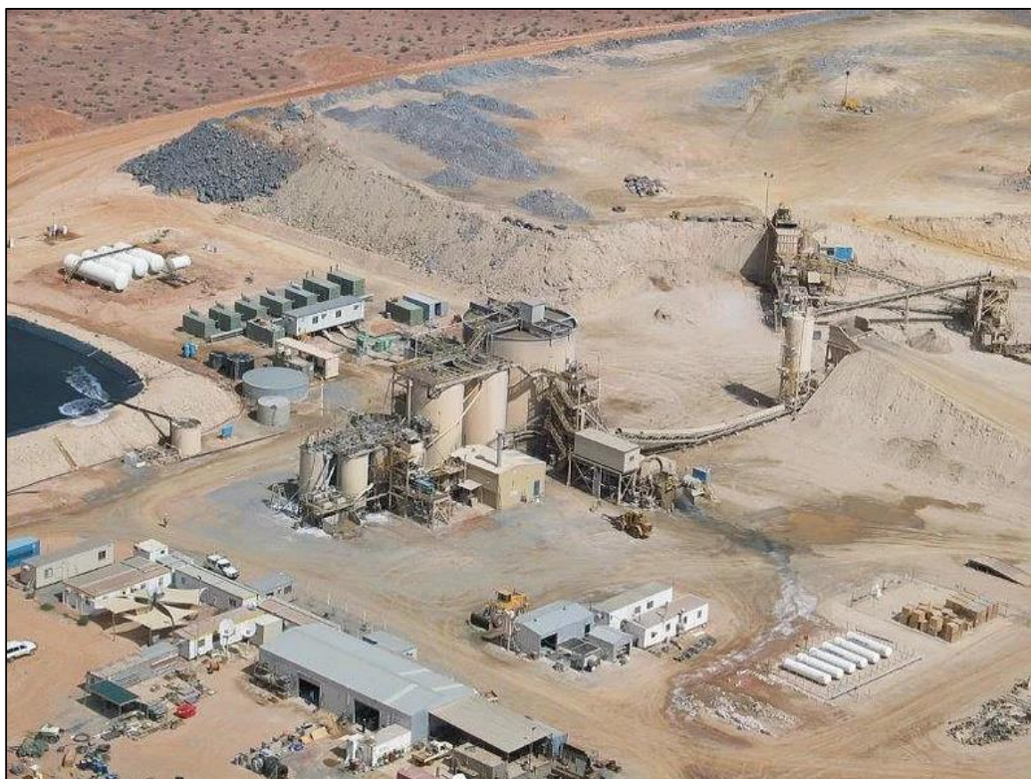
Figure 6 – Central Gawler Mill with Loading Ramp to Hopper and Ball Mill Circuit
